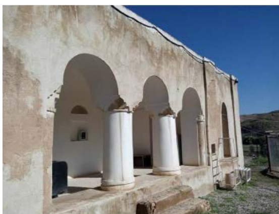
Plate 5. Right: A view of Jahangir Abad building, view from northeast; left: Entrance porch of southern side of the building (photo by Sharifinia).
