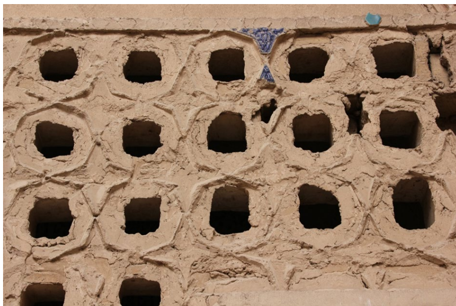
Img. 11: Detail of the grill separating the burial chamber of the Shaykh from the main space of the iwan of the Pir-i Bakran mausoleum: tile shapes and dimensions are visible on the adhesion mortar, which contains some tile fragments. (Grbanovic 2018)
