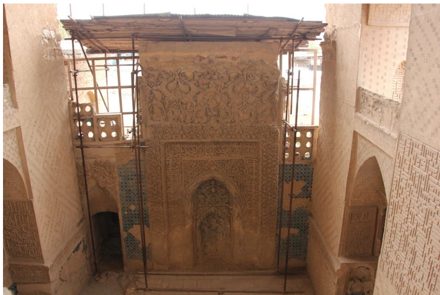
Img. 6: Stucco mihrab at the Pir-i Bakran mausoleum (second stage; 1303-04). The left and right sides of the mihrab reveal remains of separation grills which carried the perforated octagonal and four pointed tiles. (Grbanovic 2016)
