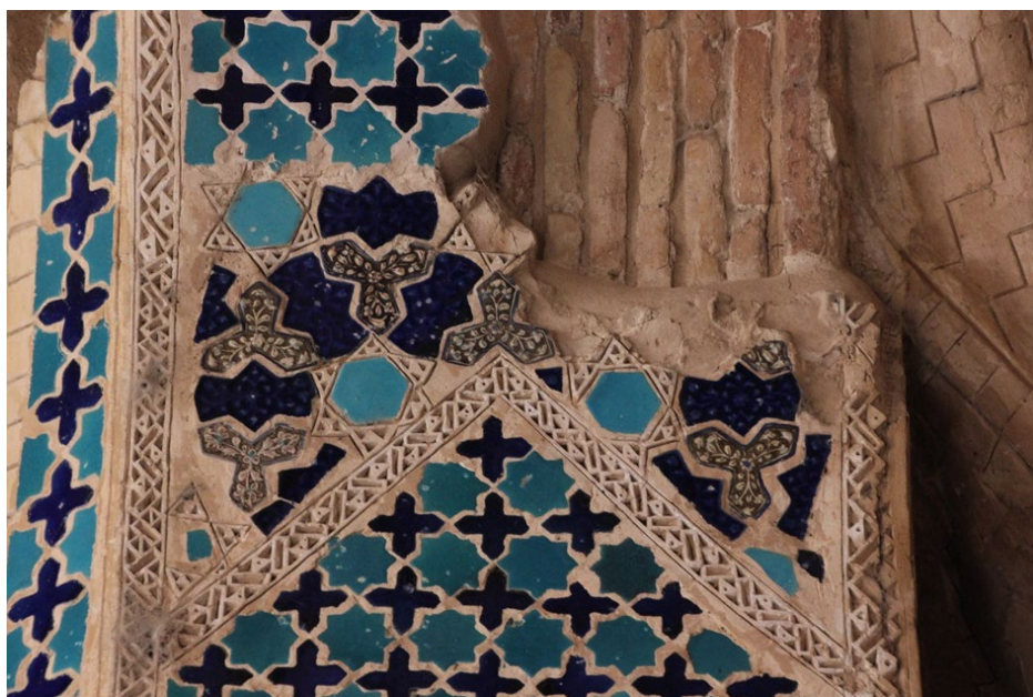
Img. 7: Luster tiles of the Pir-i Bakran mausoleum (first decorative stage) were likely reapplied on its architectural surfaces during restoration interventions. The tiles are currently located in the intrados of the iwān 's ceiling. (Grbanovic 2014)
