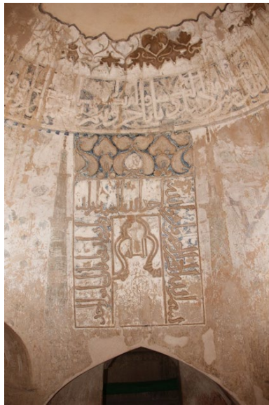
Img. 3: Wall painting and applied moulded stucco revetments at the pre-Ilkhanid domed structure of the Pir-i Bakran mausoleum are likely work of the third decorative stage. (Grbanovic 2018)
