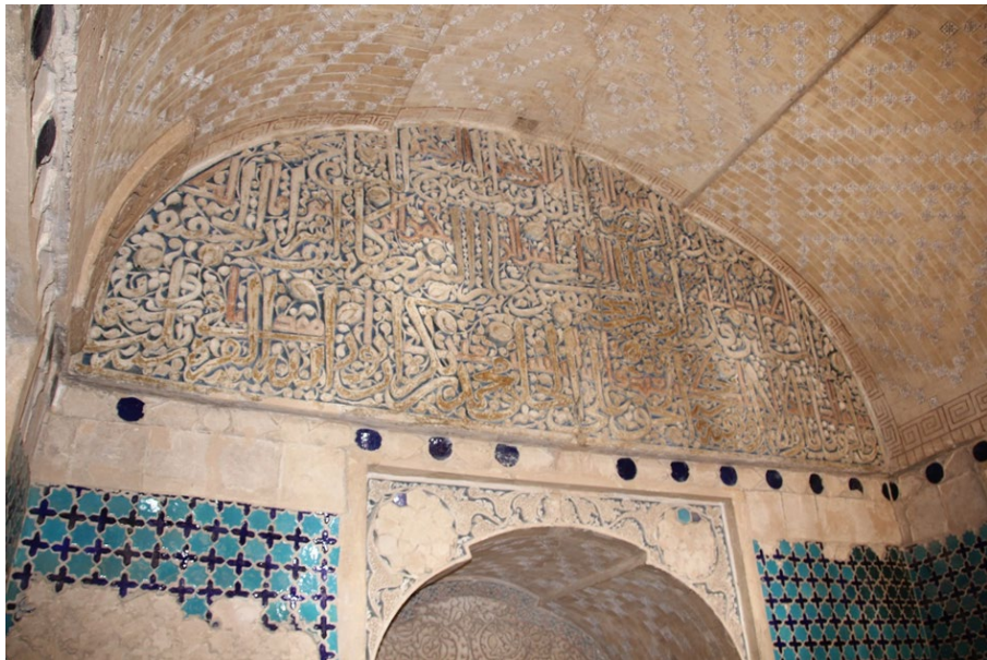
Img. 5: Pir-i Bakran mausoleum burial chamber; ceiling – the khatt-i banna'i (first stage); stucco inscription dated 1303-04 (second stage), which conceals earlier revetments in stucco and cut ceramic inscription (first stage); moulds of tile frieze from the first decorative stage; star and cross tiles (third stage). (Grbanovic 2018)
