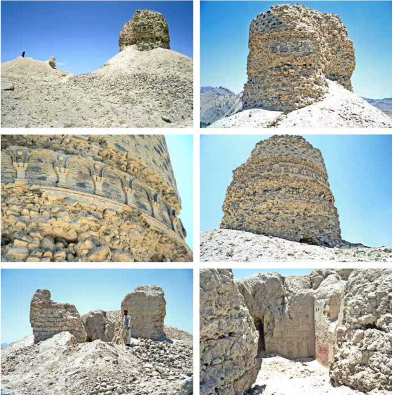
Figure 306 Wardak 1 and the remains of its associated monastery (Copyright © J.L. Lee 2003, all rights reserved)
