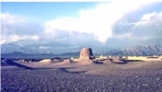
Figure 273 Hadda 10 from the south surrounded by the mounds of the courtyard chapels. Photograph: © Z. Tarzi c. 1975
