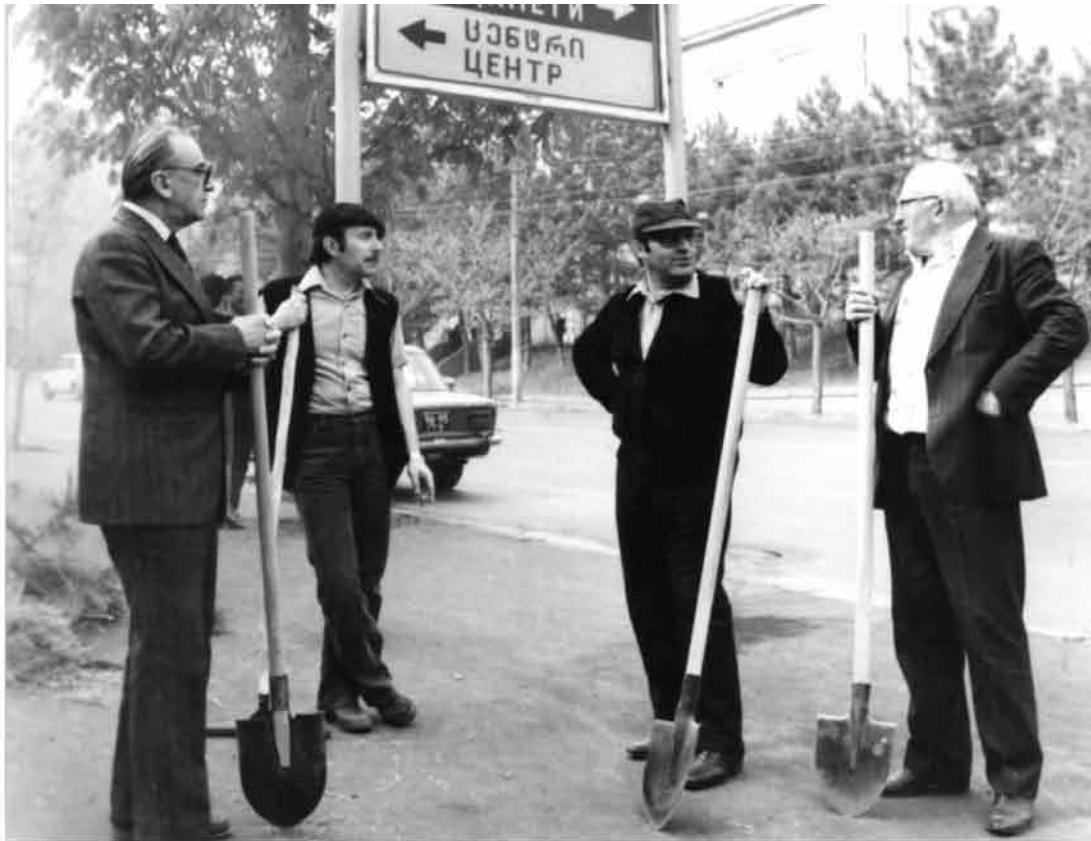
Works in the adjoining street of the Institute (late 1970s)
