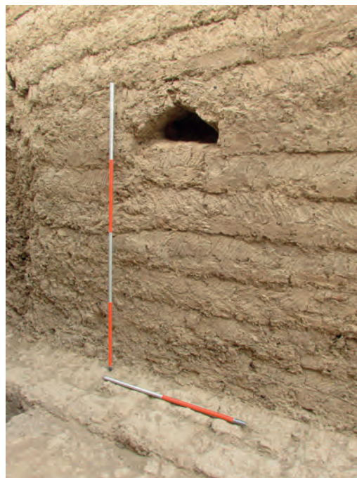
Fig. 41. The south niche in the west wall of Room 2. Note the possible bench and the right-hand jamb of the doorway into Room 3.
