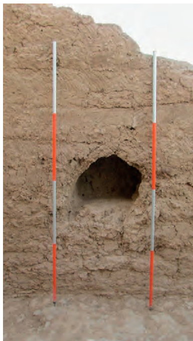
Fig. 40. The north niche in the west wall of Room 2.
