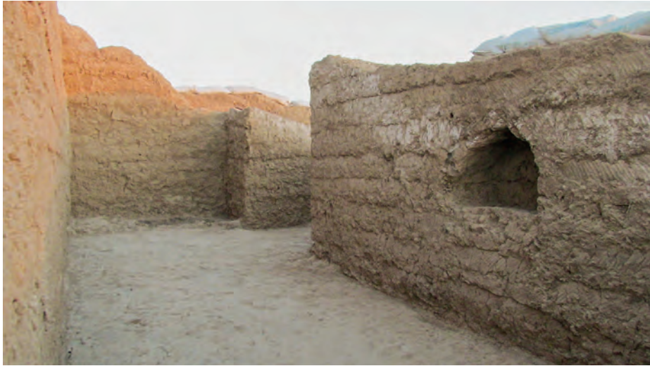
Fig. 47. Room 3 looking south showing the entrance to the west bay and the niche in the northern part of the west wall.
