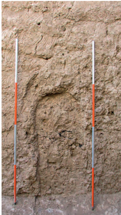
Fig. 37. The doorway from Room 2 to Room 1.
